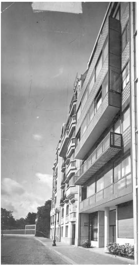
Immeuble Molitor, circa 1930 © FLC / ADAGP
