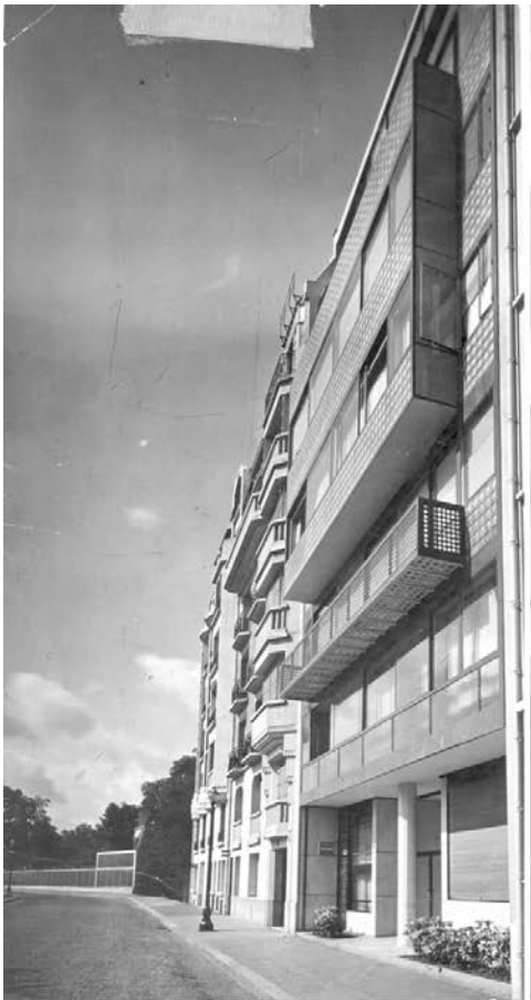
Immeuble Molitor, circa 1930 © FLC / ADAGP
